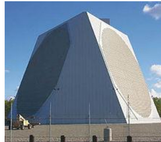
Phased array systems signal processing
