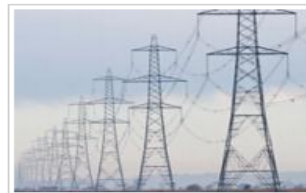
Coordinated attacks against substations and transmission lines in power grids
