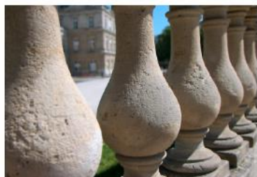
(a) I01 Stone Pillars Outside
