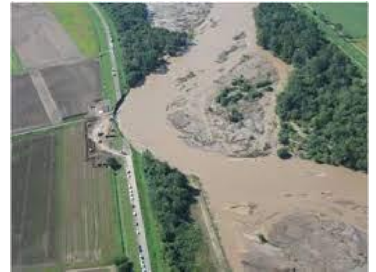
Fig.1 Bank corrosion of Otofuke River (Hokkaido, Japan) due to meandering in 2011 [1]
